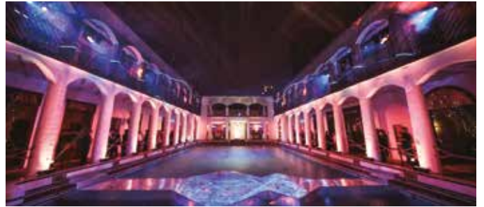
Columbia Circle, a historic compound that served as a country club for American expats from 1927-1942, has been restored and reopened as a mixed-use complex featuring F&B outlets, arts and entertainment venues and offices.
